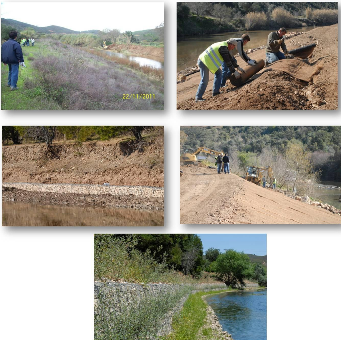
Figure 2 Pictures taken at the outset of the bioengineering works at the selected sites on the Odelouca – winter 2011 – 2012. Gabions (not a NWRM but a means to the implementation of one of them) had to be placed along the right banks at site M where (i) erosion was so intense and (ii) heavy machinery aggravated the situation that the bank was in danger of collapsing.
