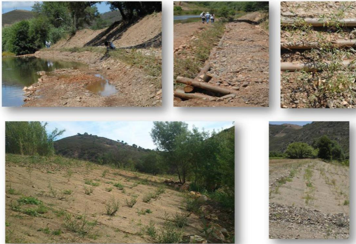
Figure 1 Examples of bank stabilisation techniques used at the Odelouca rehabilitation sites. The top photographs show the bank corrected by construction of a crib wall. The lower photographs show a bank that has been resectioned to give a more natural profile, covered with geotextile and planted with a selection of native species.
