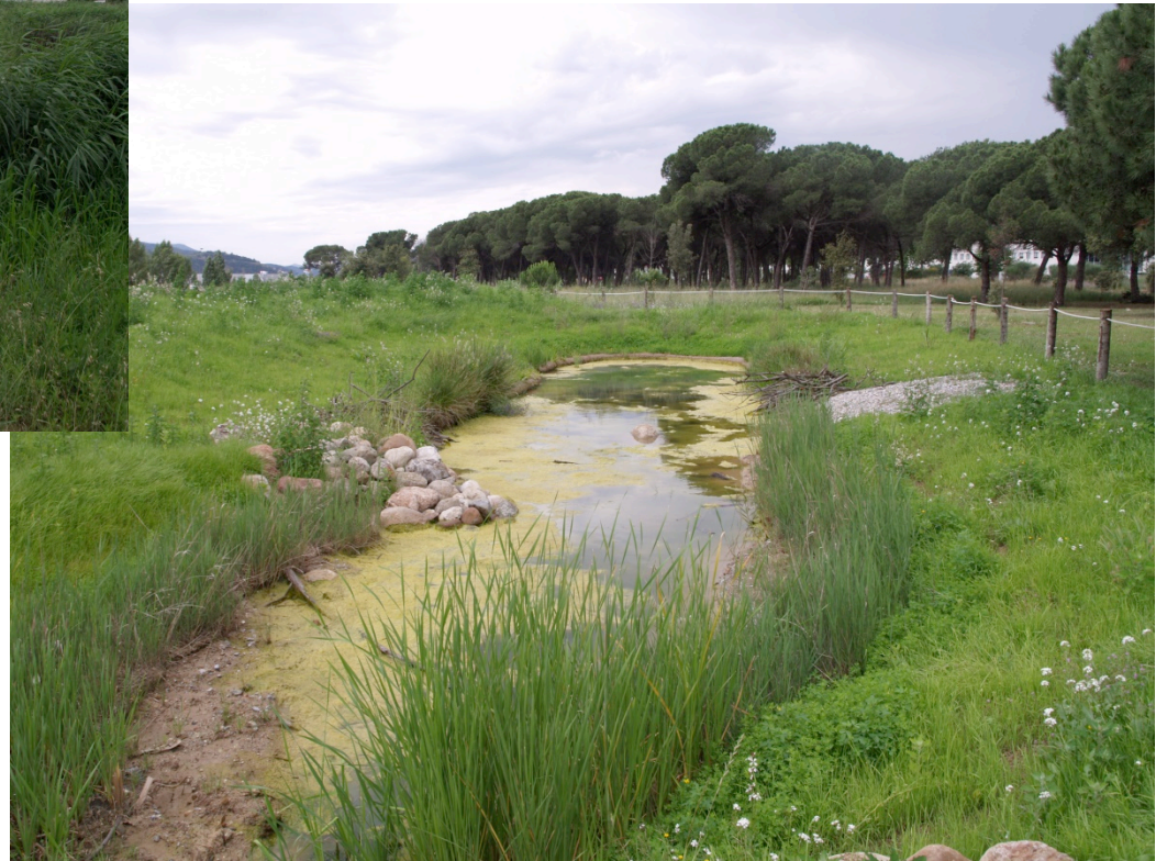
Constructed wetlands for biodiversity and tertiary treatment of urban/ industrial wastewater (Congost River, Barcelona)
