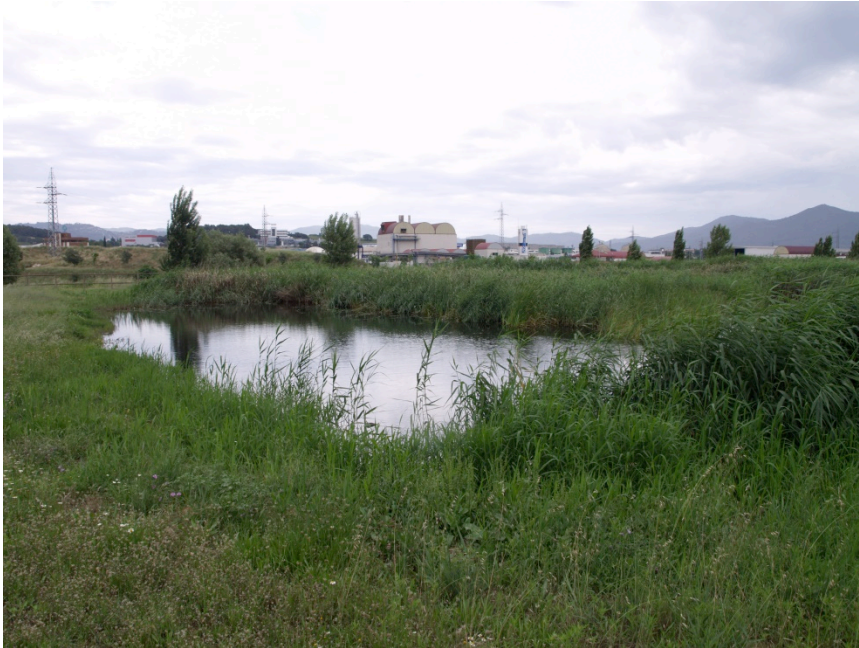
Constructed wetlands for biodiversity and tertiary treatment of urban/ industrial wastewater (Congost River, Barcelona)
