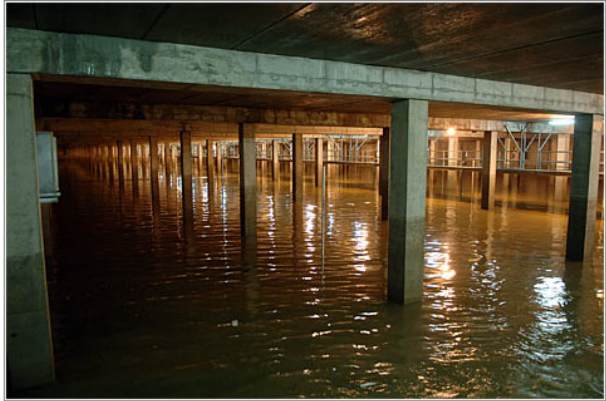
Stormwater tank in Pozuelo de Alarcón, Greater Madrid (150m long, 60m wide and 5m tall). Source: www.munimadrid.es
