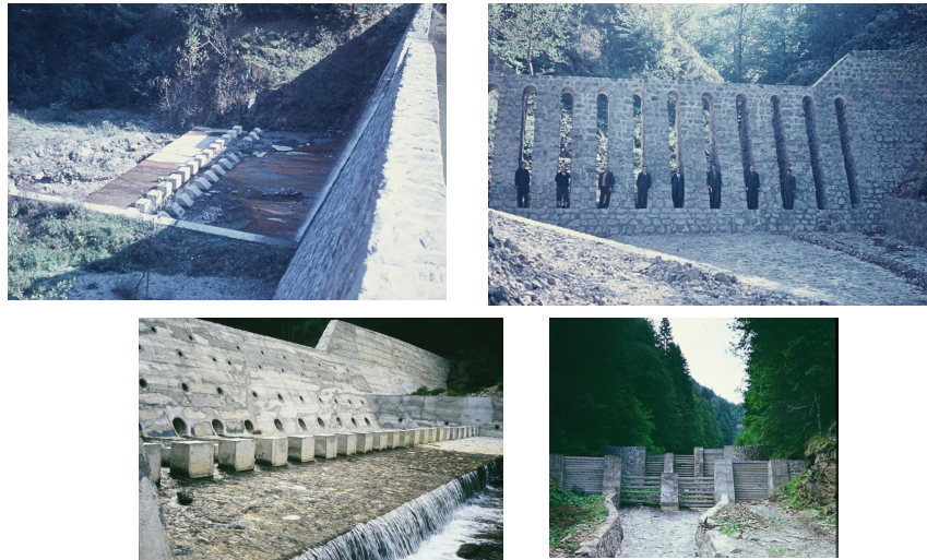
The most common dams in torrent control activity
