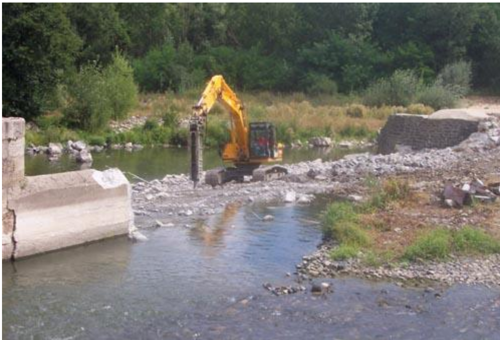
Brives dam being erased, Loire River, France
